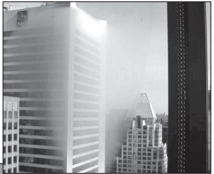
Figure 17 – Volatile fogging during a period of warm weather on a one-year-old IGU.
