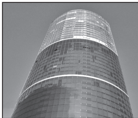
Figure 2 – Building elevation showing two-tone curtain wall.
