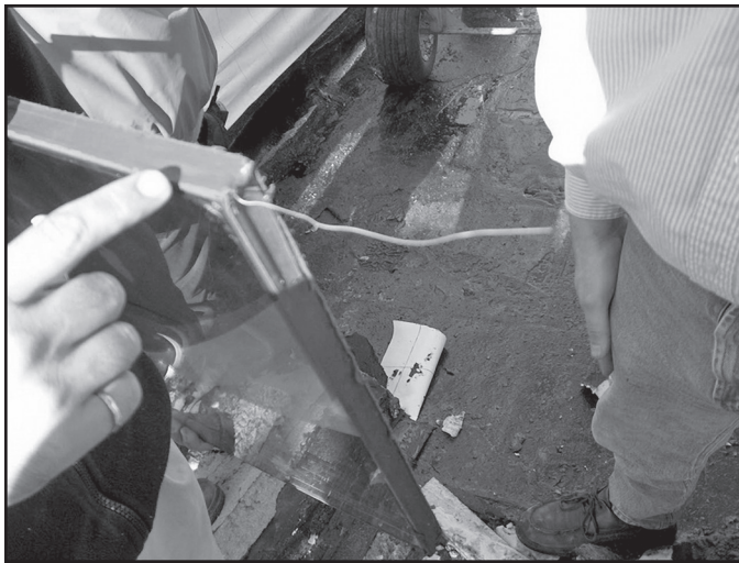
Figure 16 – The culprit was unsealed capillary tubes concealed within the window assembly.
