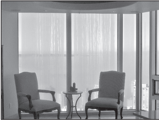
Figure 3 – Significant IGU condensation visible from the interior.
