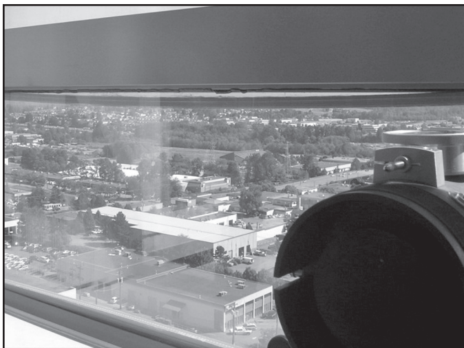
Figure 13 – Displacement of spacer bar and seal into vision area after 10 years in service.
