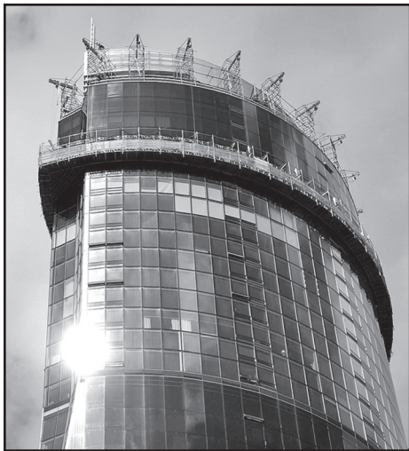
Figure 8 – High-rise tower showing a portion of the completed IGU replacement and the custom suspended scaffolding ring.
