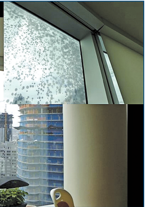
Figure 5 – Example of glass fogging in conjunction with low-E corrosion.
