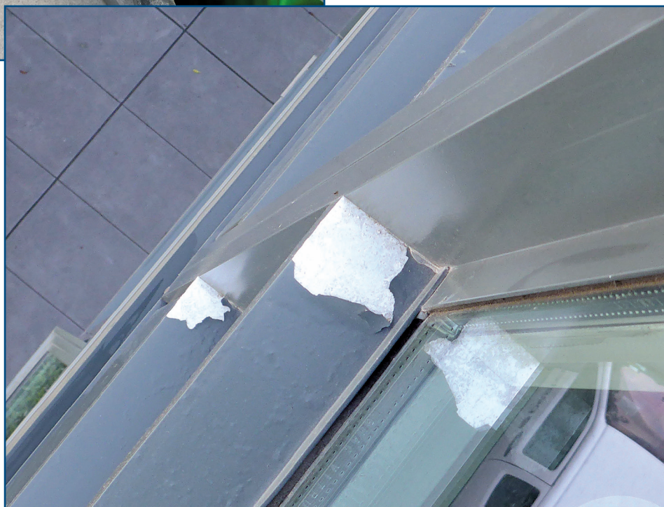
Figure 13 – Example of paint failure.
