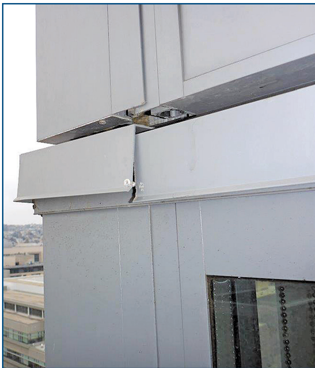
Figure 11 – Sample of trim cover failure.
