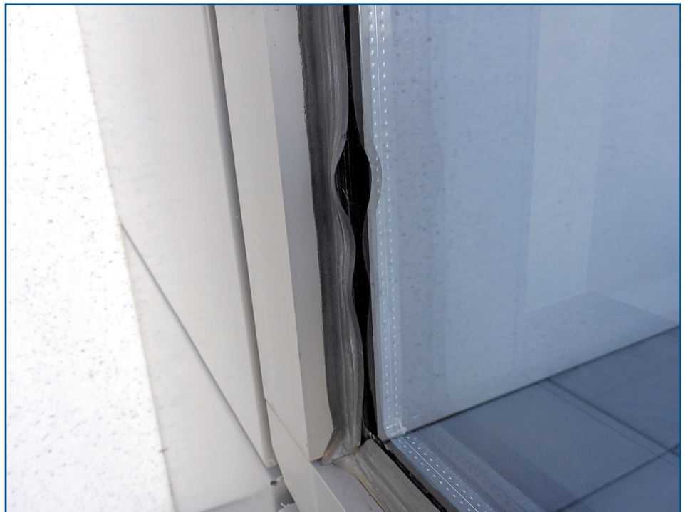
Figure 3 – Example of gasketing failure.
