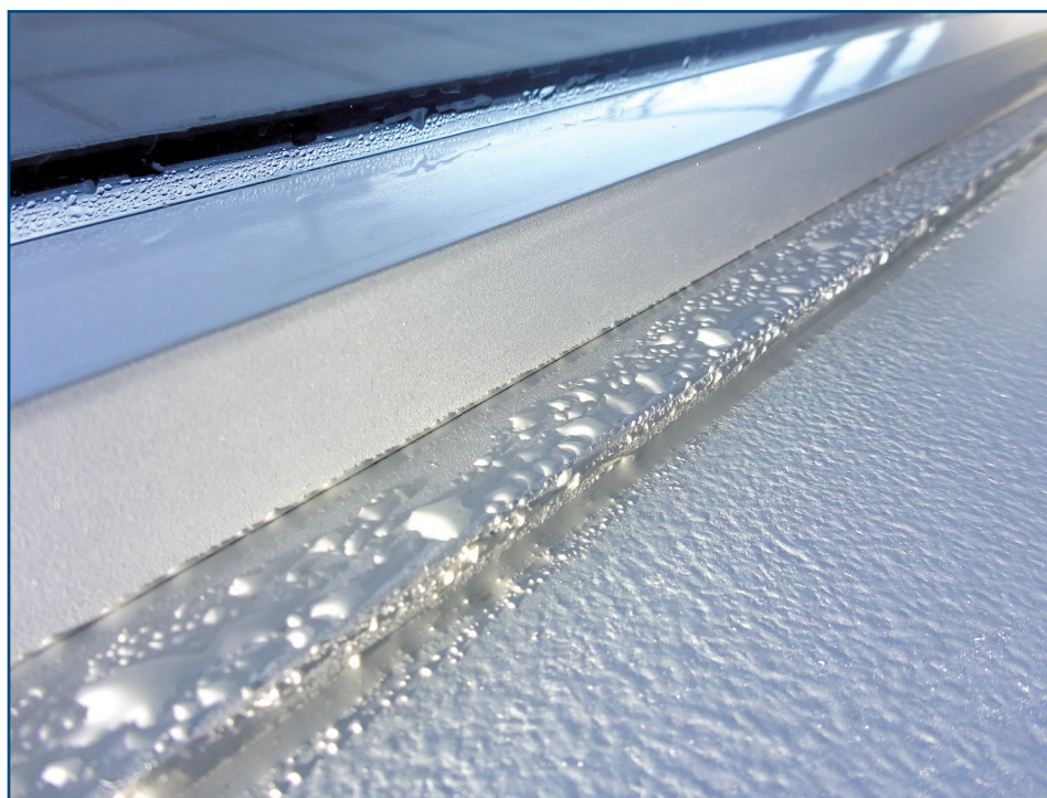
Figure 10 – Condensation on an interior window surface.
