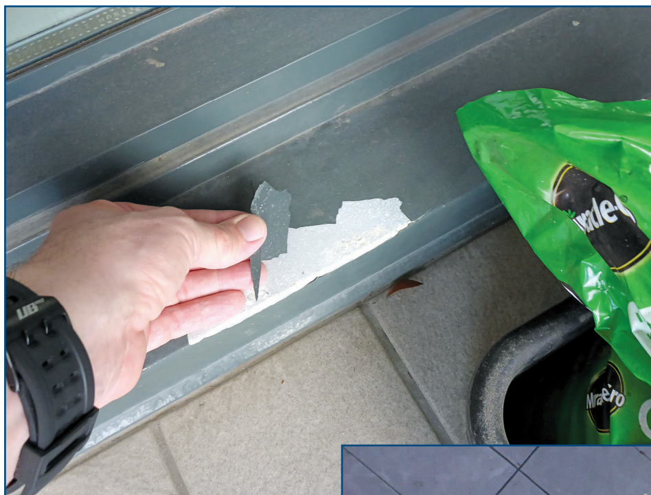
Figure 12 – Example of paint failure.
